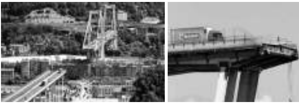
Figure 8 Genoa, August 2018 – Morandi bridge collapse
