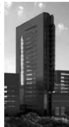
Figure 13 – Enameled panels as external cover of a building
