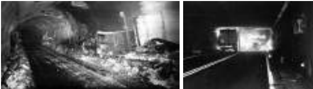
Figure 14 – Mont Blanc - 1999 - Fire in the highway tunnel
