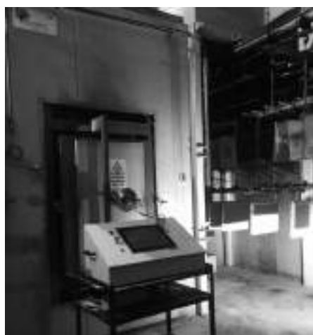
Figure 2: Industrial furnace atmosphere monitoring in Electrolux Forli plant by HELIOS MAGMA gas analyzer.
