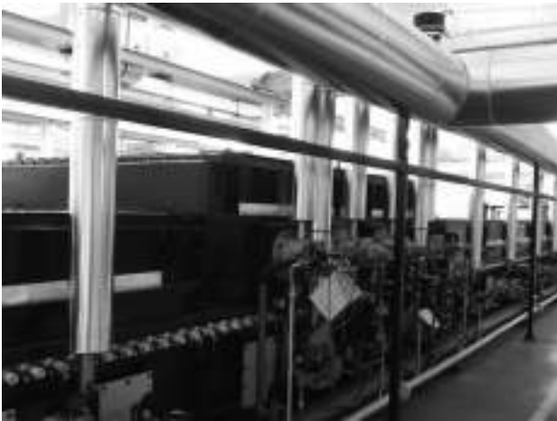
Double-heating zone in a gas-heated furnace
